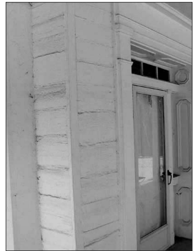
Shiplap siding on southeast corner.
