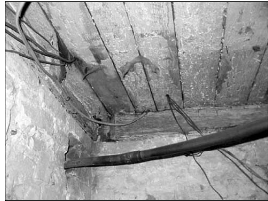
Hewn sills in cellar.
