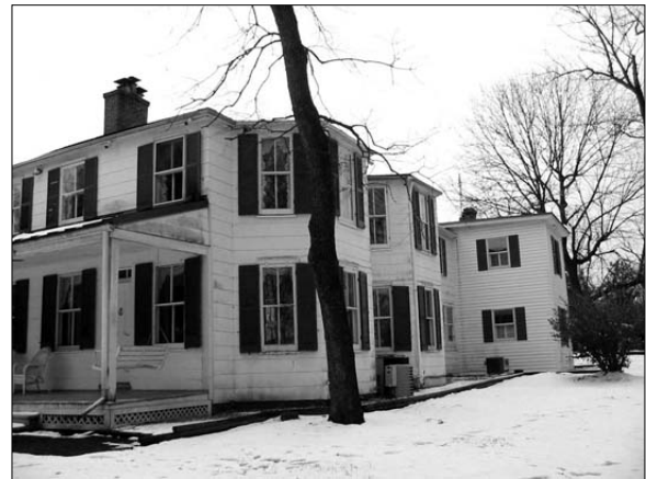
North and east elevations of house showing bay windows that were added circa 1890-1920.
